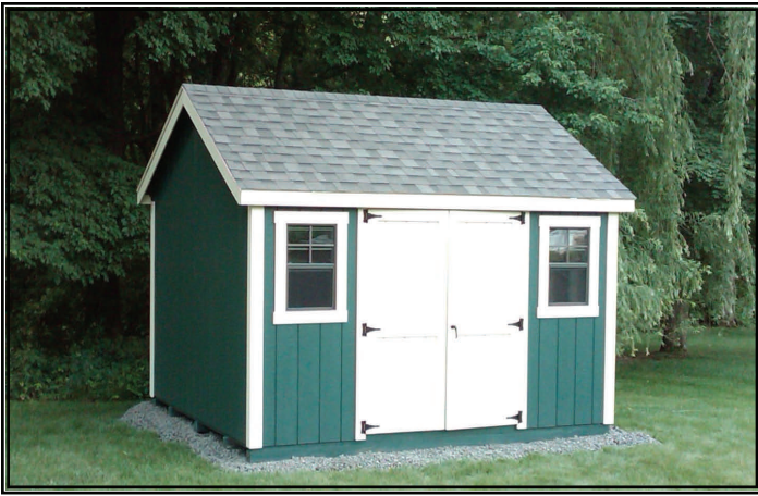
Standard Crushed Stone Pad
