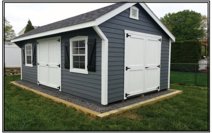
Crushed Stone pad with 1 Layer 6x6 perimeter
